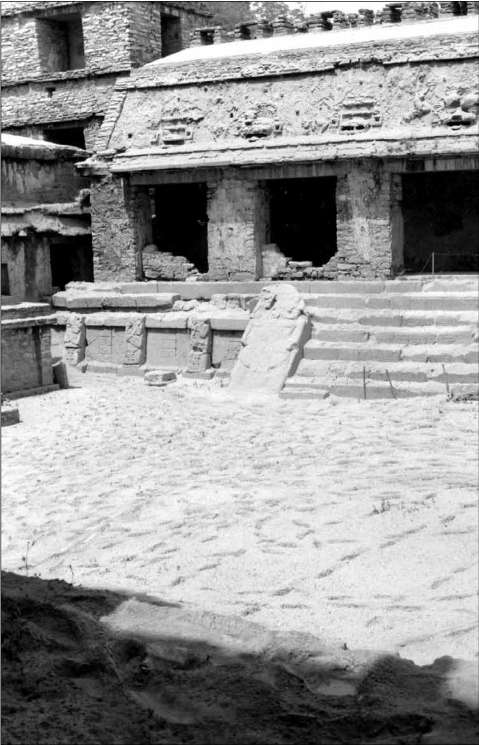
Ashfall on House C in the Palace
