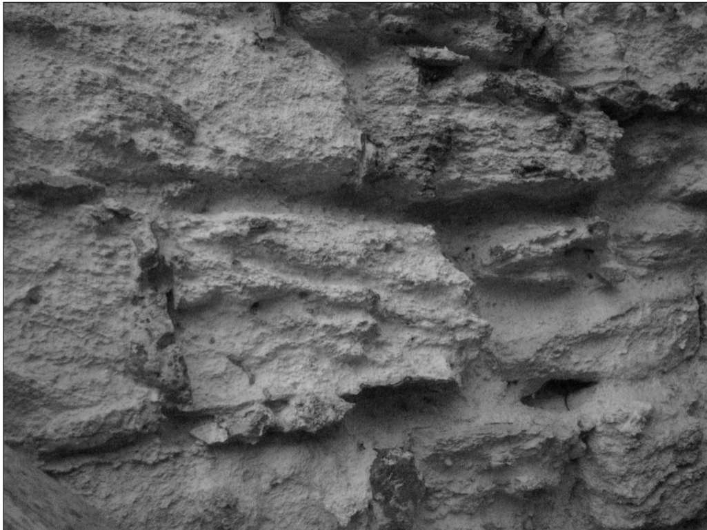
Figure 5. Damage from natural sources: eroded stone wall at Tikal (photo: J. Crasborn, 2010).
