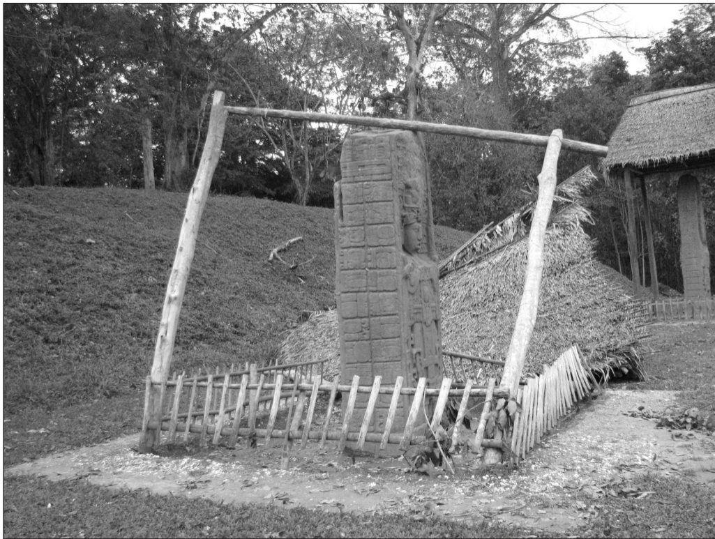
Figure 10. Hurricane damage from April, 2010, caused by the collapse of the thatch shelter over Quirigua Stela A (photo: J. Crasborn, 2010).
