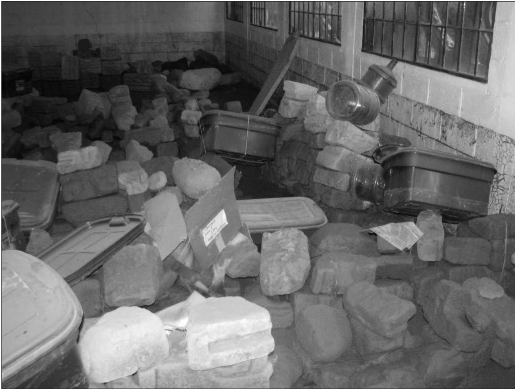
Figure 12. Damage caused by Tropical Storm Agatha in the storage building constructed in 2000 (photo: by J. Crasborn, 2010).
