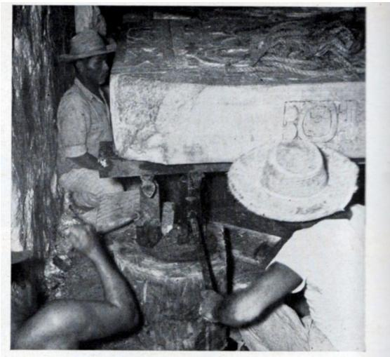
LIFTING SLAB, workers carefully turn truck jacks. Under this slab was a second heavy stone lid that also had to be raised.
