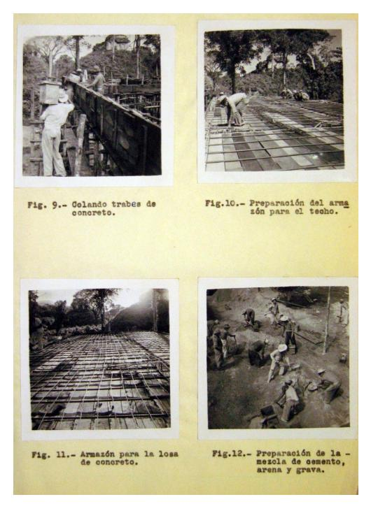
**Figure 8.2** Photos of Construction Work for the Camp Building Performed in 1950 (Source: AMNH Archives - Ruz 1950)
