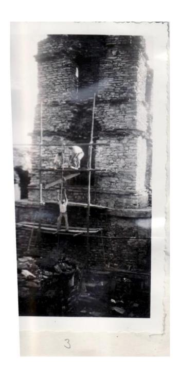
Figure 2.3 The tower as workmen brought up wooden beams to support the door frames
