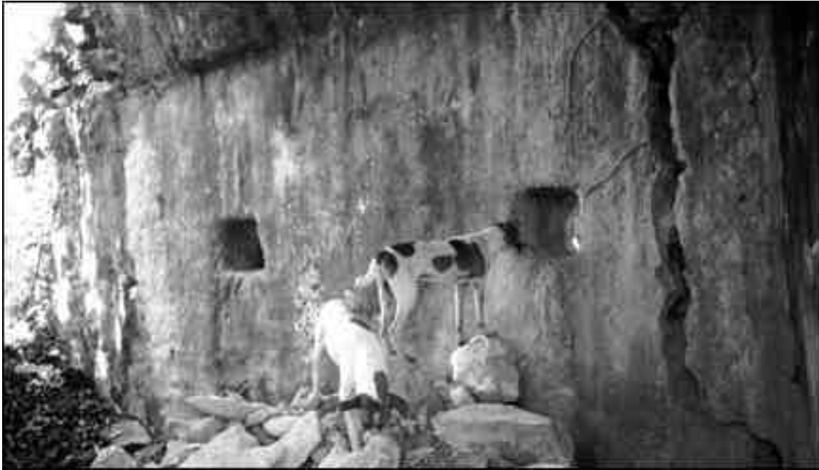
Figure 6: The back wall of Structure 1 with cracks.
