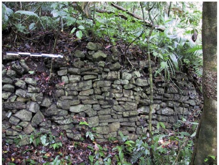
Figure 4. Year 2000 photo of an intact terrace segment in the Encantado Group.
