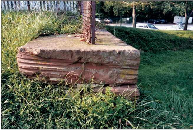
Figure 4. Rope grooves on downstream corner of Rileys Lock #24, Maryland (photo by Ron Canter).
