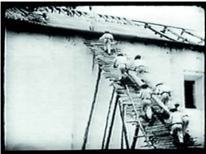
Figure 4: A large beam is being carried up the ladder; six men carry the beam while a seventh appears to be directing them. Frame from Men, Mules, and Machetes (courtesy of the Middle American Research Institute, Tulane University).
