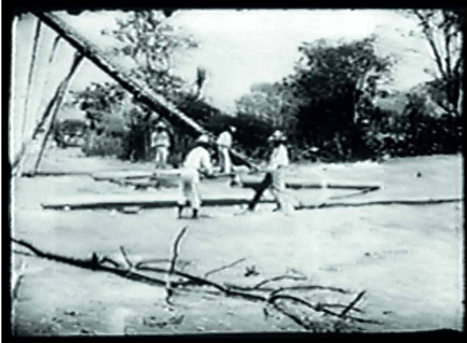
Figure 3: Motion picture frame from Ocosingo showing the ladder in the background while two men are preparing one of the beams that will be used in the renovation of the roof of the church. Frame from Men, Mules, and Machetes (courtesy of the Middle American Research Institute, Tulane University).
