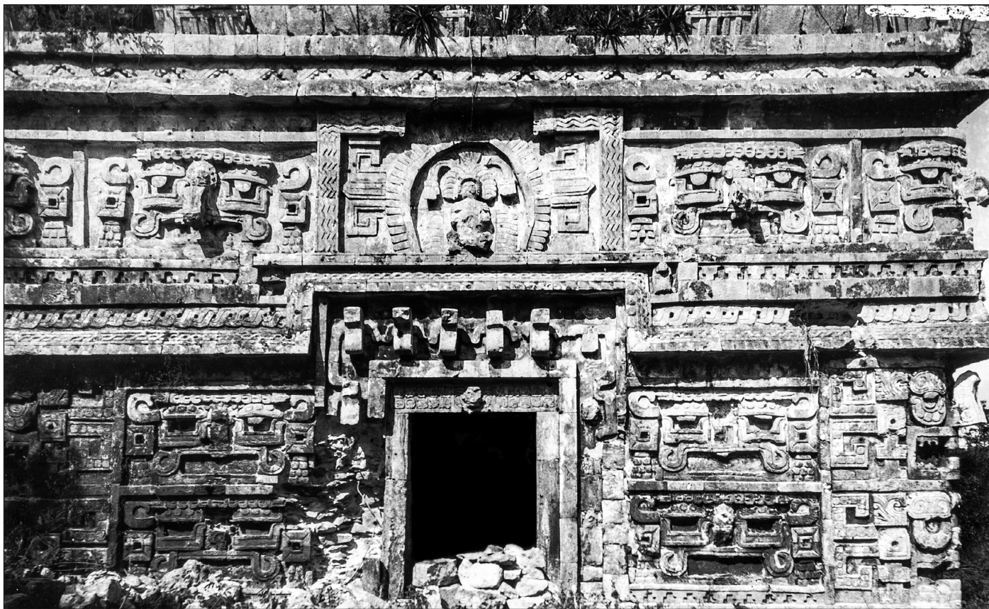
Figure 1. The east face of the East Wing of the Monjas, Chichen Itza. Photograph by Augustus Le Plongeon, probably 1875 (Lawrence Desmond, personal communication 2014), from the Lawrence G. Desmond Collection of Augustus and Alice Dixon Le Plongeon photographs. The George E. Stuart Collection of Archaeological and Other Materials, 1733-2006. Collection Number 05268. The Wilson Library, University of North Carolina-Chapel Hill.
