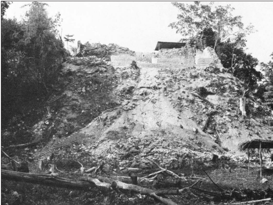
Fig. 6 Caracol Structure A3 during consolidation.
