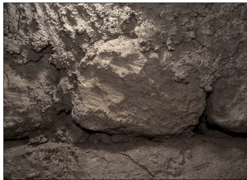
Figure 2.16. Flake scars left by masons on chamber stones. Photo: Arturo Godoy.
