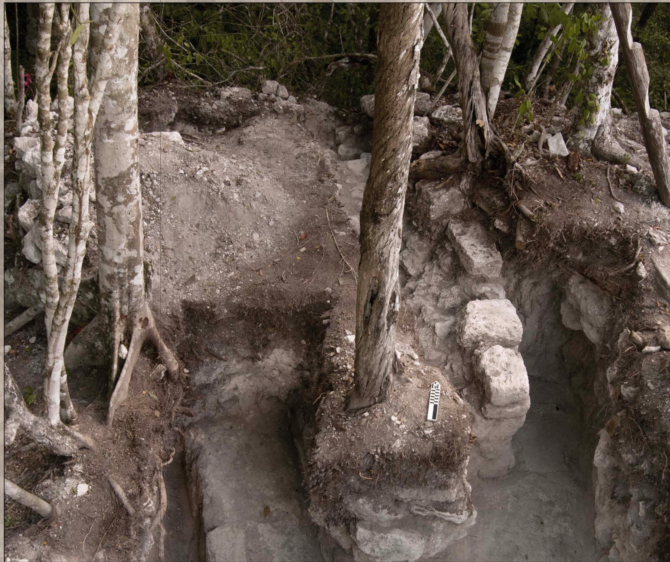
Figure 2.1. Summit of the F8-1 pyramid with remains of the final construction phase, Str. F8-1-1 a . Photo: Arturo Godoy.
