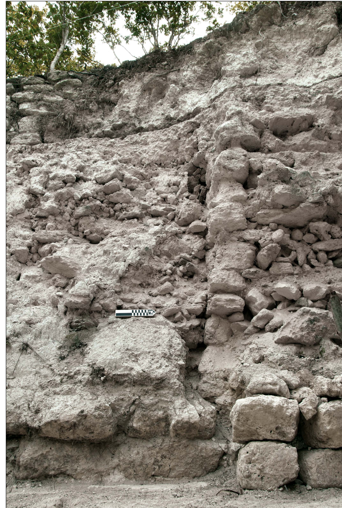
Figure 2.47. Fill above the Temple of the Night Sun, with retaining walls to prevent lateral displacement of the newly added bulk for Str. F8-1-2 nd . Photo: Arturo Godoy.
