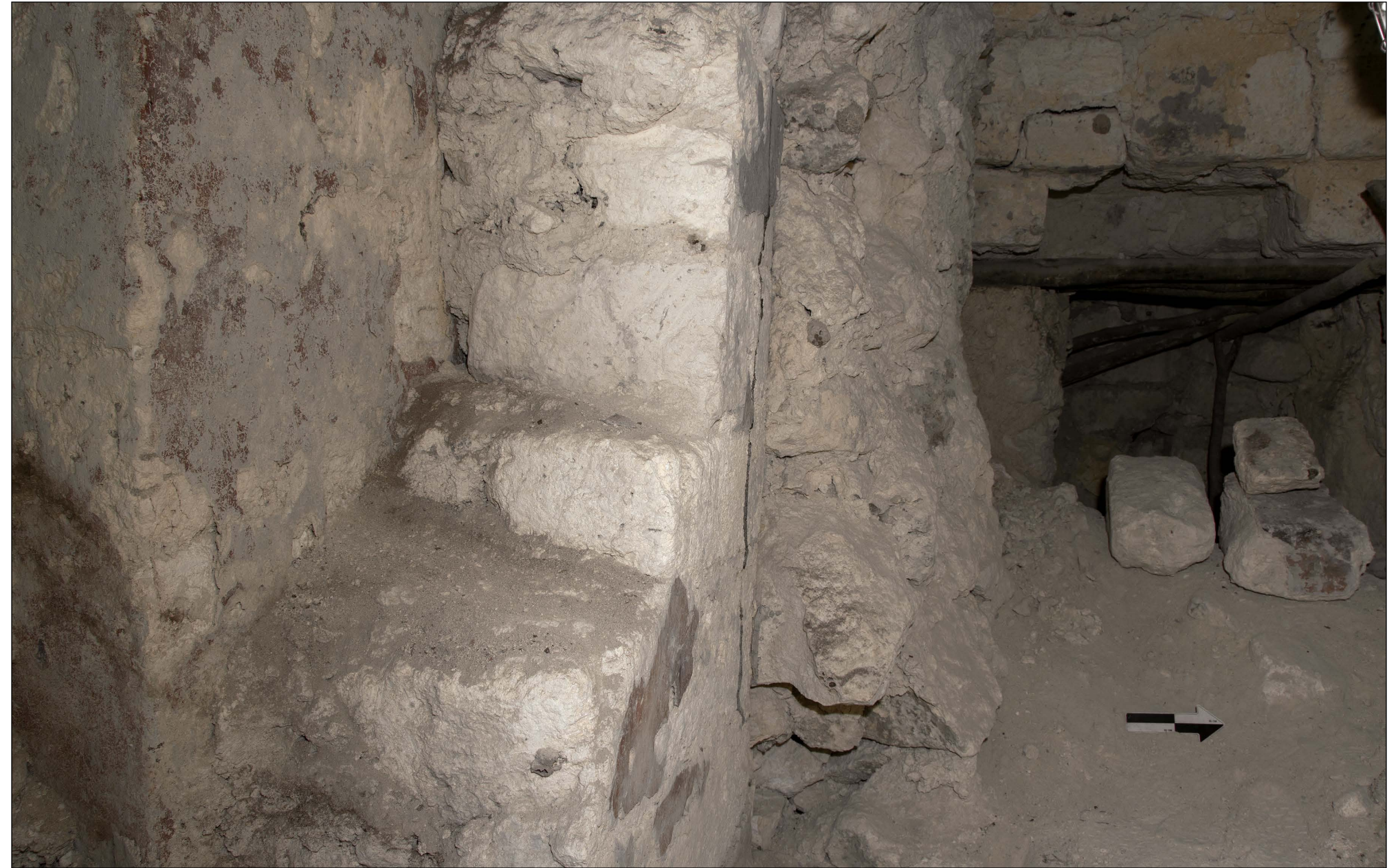
Figure 2.30. Front chamber of Temple of the Night Sun, reinforced by thickening the door jamb of its middle wall to combat structural failures. Photo: Arturo Godoy.
