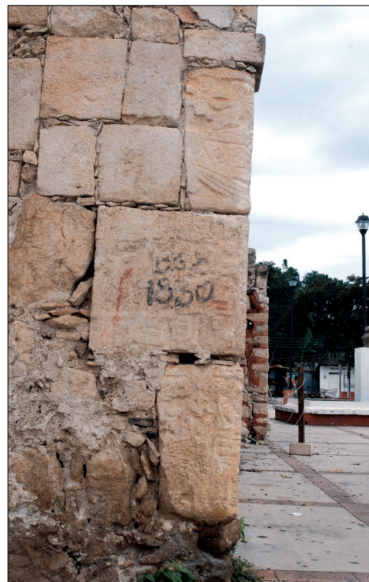
Figure 8. The small chapel in Piste (Yucatan) has a large number of sculptures and reliefs from nearby Chichen Itza embedded in its exterior walls and façade. Several can be seen on the corner here (photo: Christian Heck).
