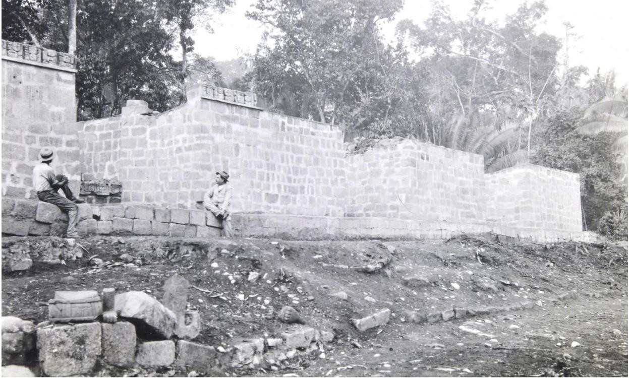
Figure A.25. Two unidentified men sitting on the platform of the restored Structure 1B-1 at the end of the 1912 season. Note the placement of the cornice hieroglyphic frieze. Within the first of the three doorways the hieroglyphic bench is visible. Also note that the interior wall facing the hieroglyphic bench has been reconstructed despite its originally still having its stucco surface finish (see Figure A.19 above).
