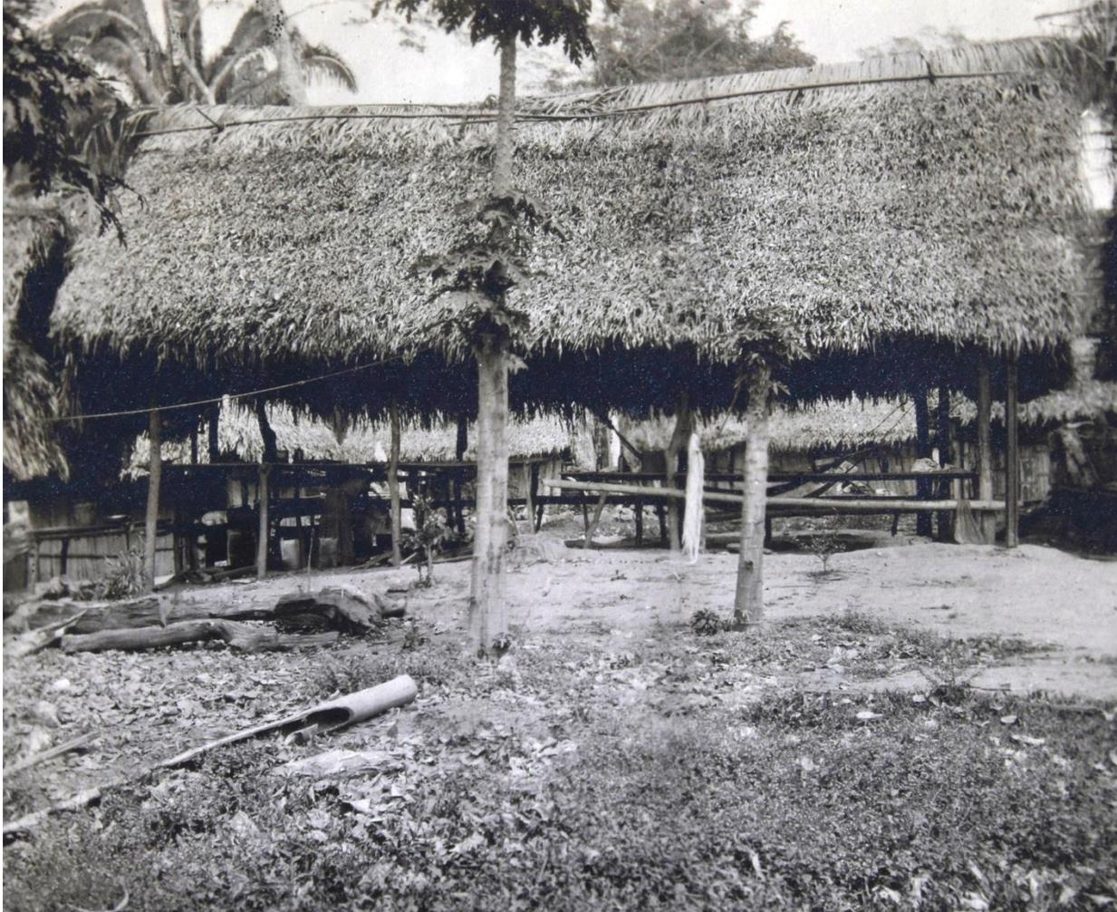
Figure A.10. A photo of the field camp, which consisted of a series of corozo or manaca palm-roofed *champas*, or huts. The field kitchen is in the background to the left. This kind of structure was ubiquitous throughout the Maya lowlands, especially along the trails used by *chicleros* and *mulada arrieros*.
