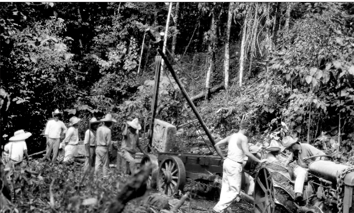
Removing monument with makeshift pulley and tractor (Piedras Negras Archives unnumbered).
