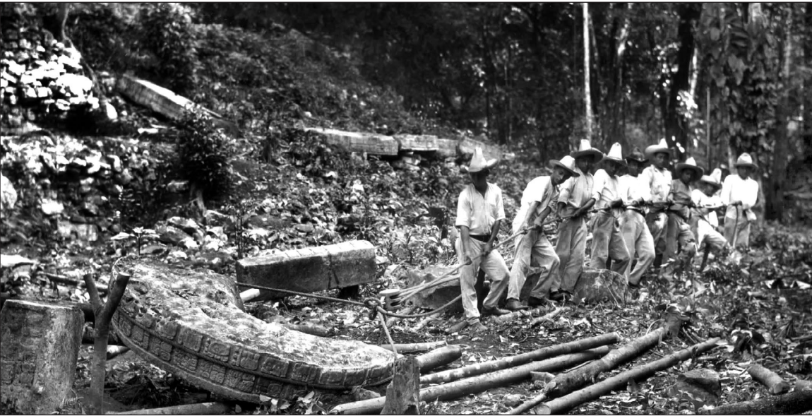
Laborers moving a fragment of a circular monument (Piedras Negras Archives unnumbered).
